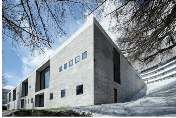
Figure 4. Therma Vals, designed by Peter Zumthor, is appreciated by other architects, architectural critics and architectural media for its reciprocal relationship with its site. The scale of the building reinforces this relationship by allowing it to be embedded in the sloping topography of the site (Arkitektur, 2025).
